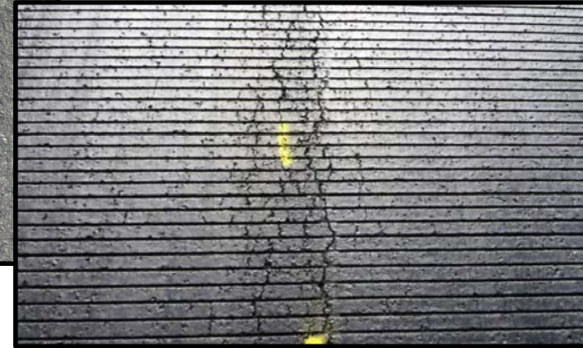
Top-down cracking
